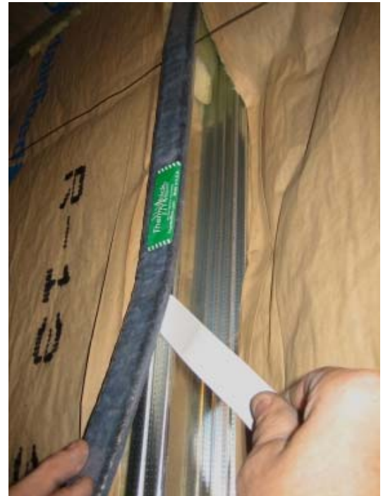
Simple Peel and Stick Adhesion to Metal Framing for Low Cost Installation
