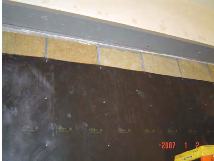
View of Acoustiblok® Added to Metal Studs
