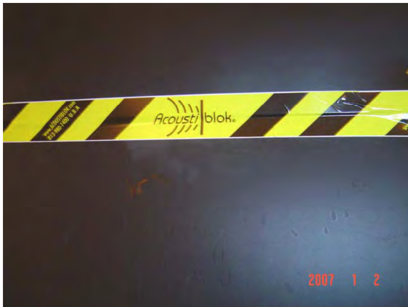
View of Acoustiblok® with Acoustigrip® Tape at Seams
