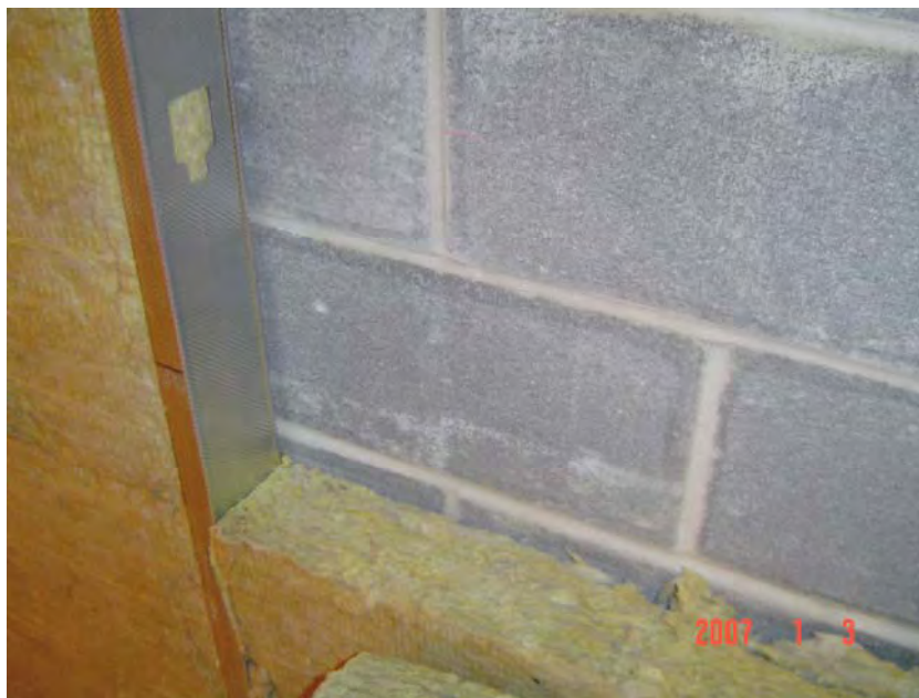
View of Metal Studs with Insulation and 1/2" Air Space
