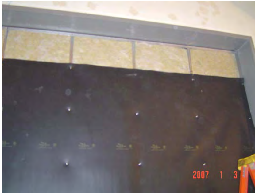
View of Acoustiblok® Added to Metal Studs
